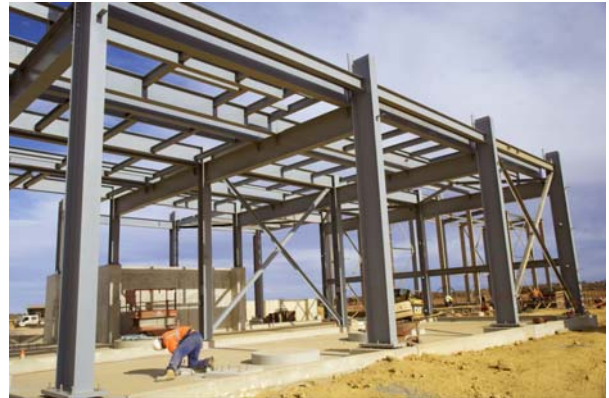
Concentrator Construction Progress
