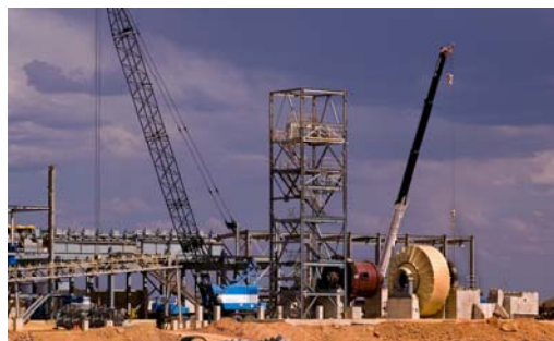
Construction at Jaguar
